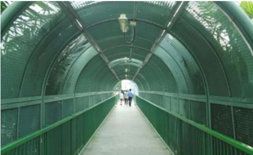
See through fencing covering a predictable route provides visibility
